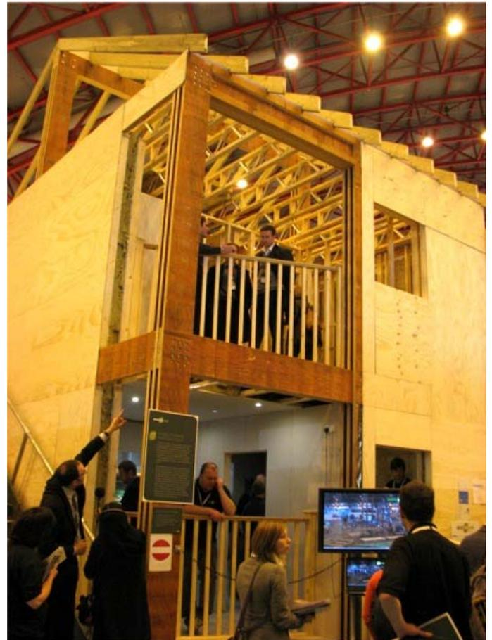
**The Zero Carbon House - in cut away view of course so that it is possible to see how it is all done. To see a time lapse video of it being constructed go to [www.ruralzed.com/video.php](http://www.ruralzed.com/video.php)**
